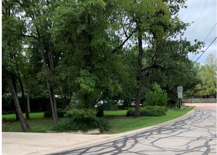
West Roadside Ditch of Sunset
