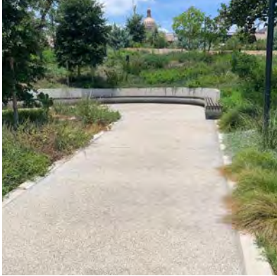
1 11' Pervious Concrete Multiuse Trail
