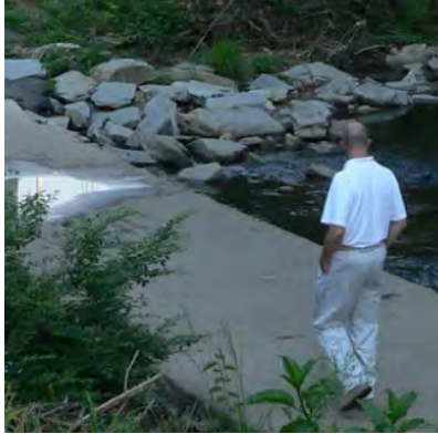
3 11' Concrete Low Water Crossing
